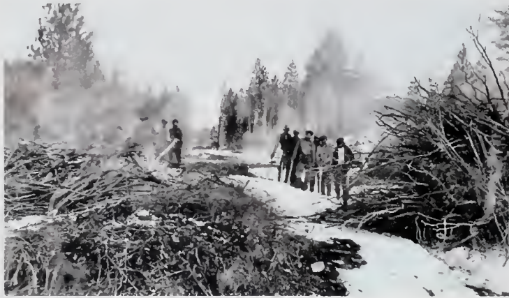
Clearing brush to build roads.
